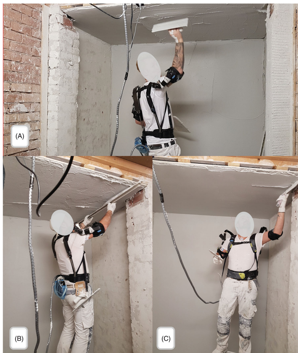
Figure 1. Overview of the set-up and activities on the ceiling. (A) applying the gypsum to the ceiling, (B) screeding and (C) finishing with a plastering spatula.
